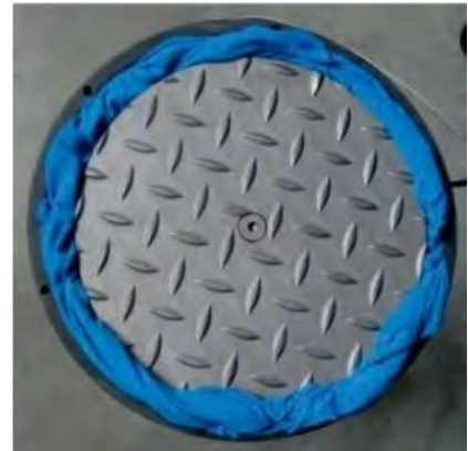
Figure 5.6 - Sealing the bollard
